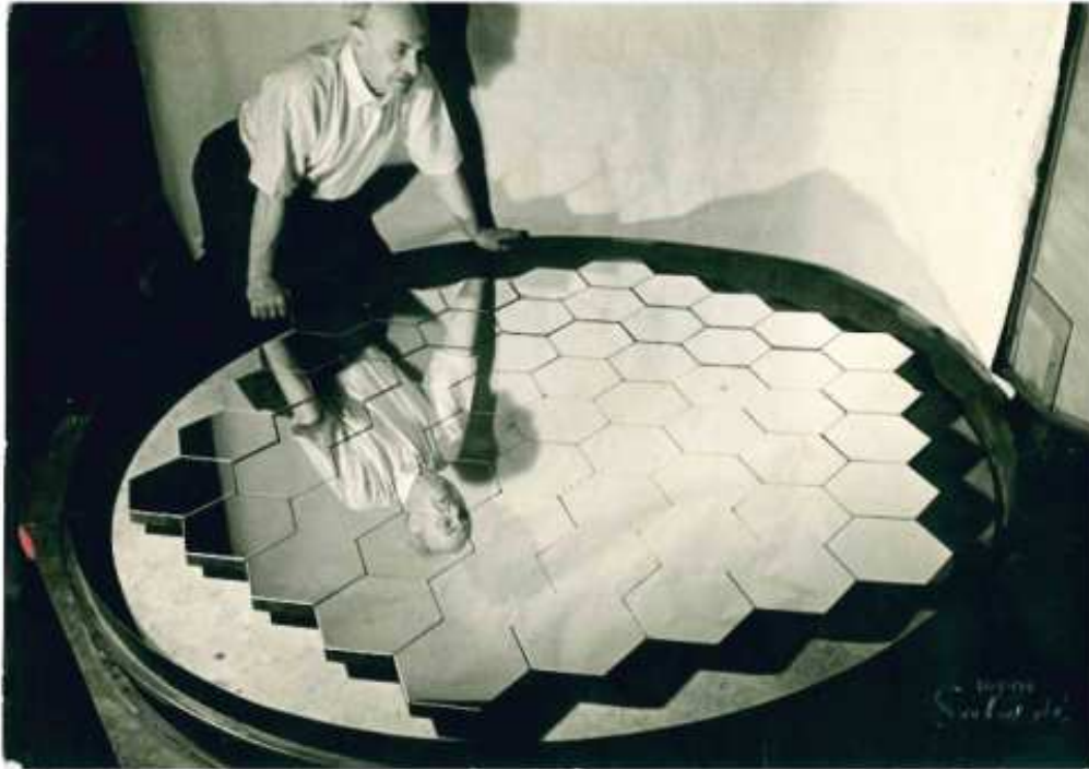
Fig. 8. Summer 1952: Horn d'Arturo admires the completed 1.80 m tessellated mirror. (HORN D'ARTURO 1955)
